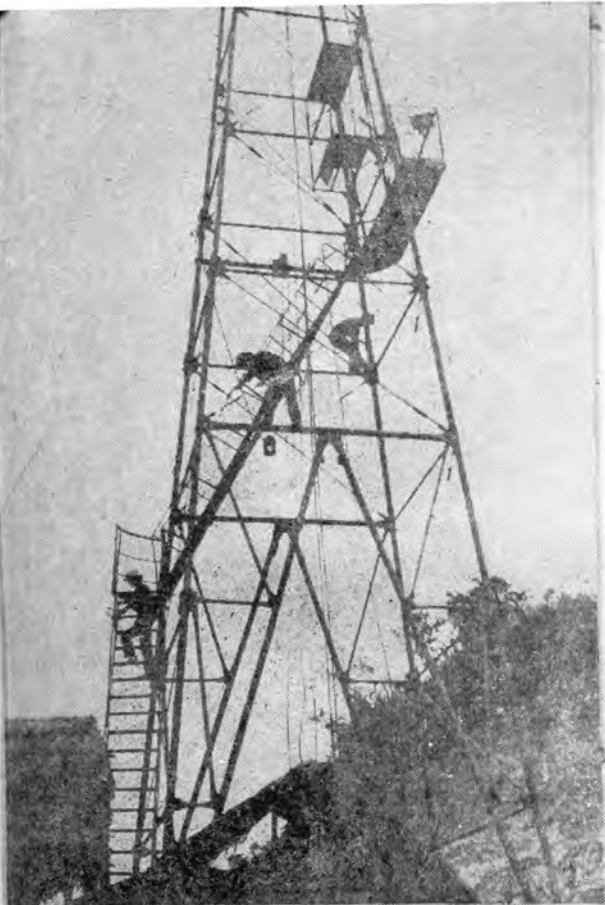
Erecting a drilling-rig.
