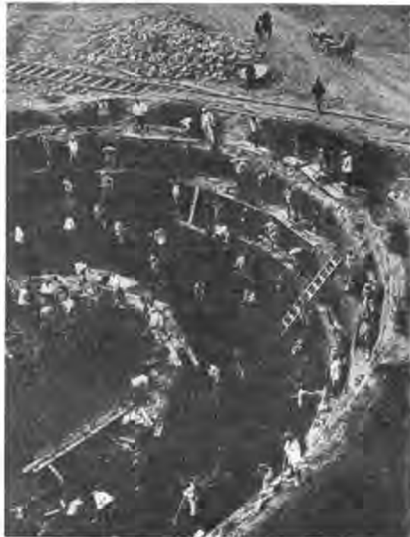
Digging the foundation of a blast furnace at Magnitogorsk.
