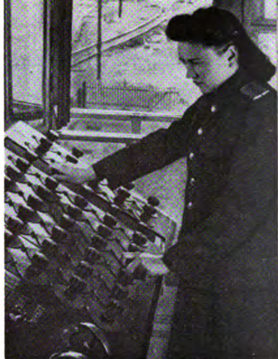
AUTOMATIC YARD CONTROL. Above: An operator in a mechanized hump yard moves switches by remote control. Left: A train marshaled automatically.
