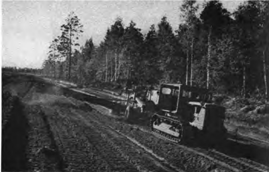
ROAD BUILDING. New roads are appearing rapidly throughout the Kuibyshev project area. A powerful grader at work at the development site.
