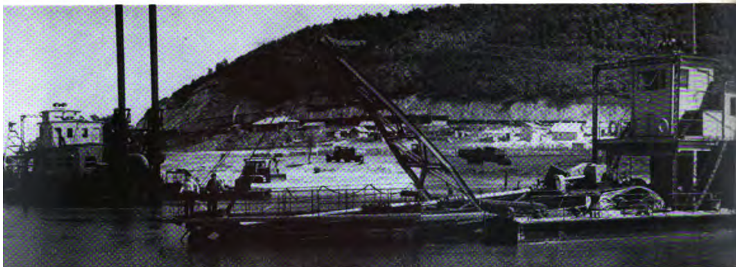
Suction dredges at work filling earthen dams and dikes at the Kuibyshev development.
