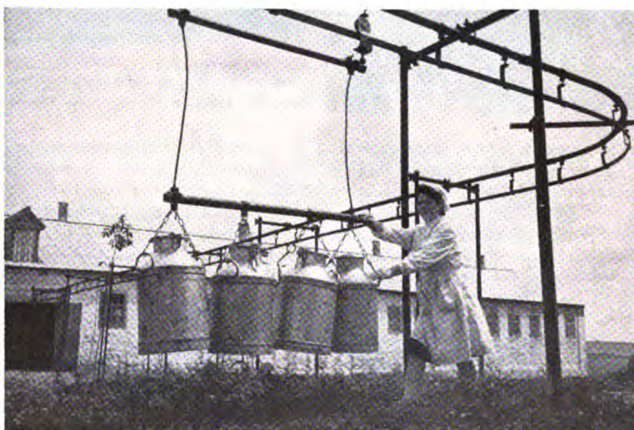
MECHANIZED DAIRYING. Introduction of labor-saving devices on Soviet farms is making great progress. Above: Moving milk cans by suspension railway.
