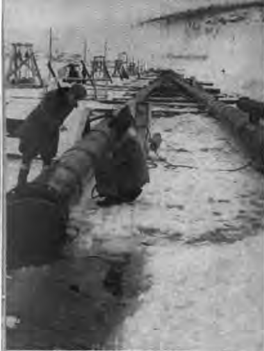
PIPELINE. Half a mile long, the pipe will transport sand across the Volga.
