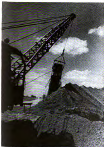
EXCAVATOR. An OM-202 electric dragline at work on the canal of the lower lock at Kuibyshev.
