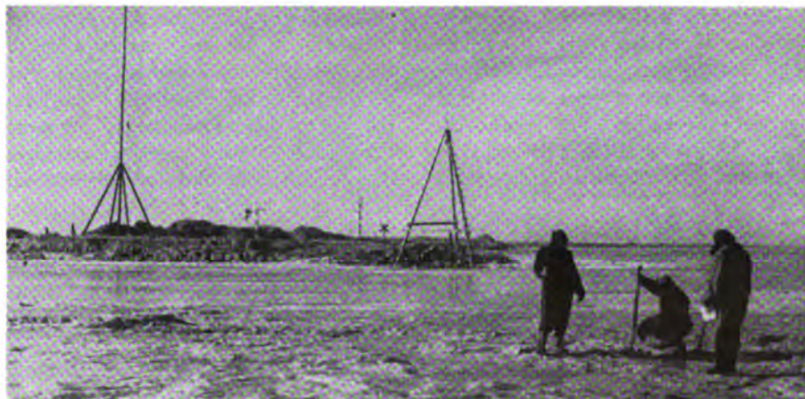
SURVEYING THE AMU DARYA. Complete information about the river's behavior in all seasons must be gathered. Hydrologists measure the depth of winter ice.
