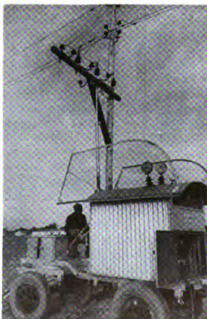
ELECTRIC MACHINES. Tractors operating by local electric power conveyed by reeled cables are used on many fields in the USSR. A mobile transformer sub-station (left) and an electro-tractor on the cotton fields of the Communist Collective Farm, Uzbek SSR.
