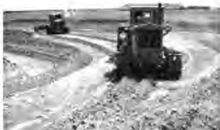
RESERVOIR SITE. Tractor-drawn excavators at work on the site of the reservoir of the Trudovik Collective Farm, Rostov Region.
