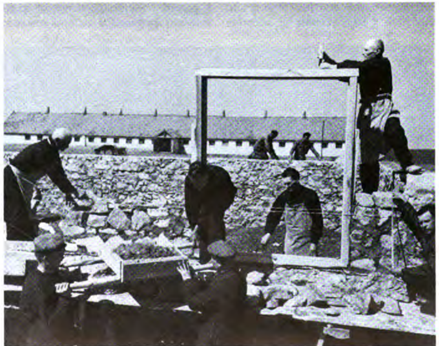
BUILDING A CATTLE BARN. A brigade of workers erecting walls for the structure on the Pobeda Collective Farm.
