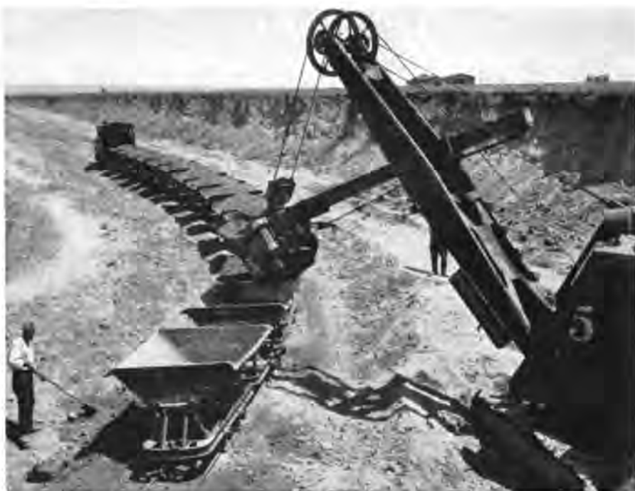
CONSTRUCTION IN ROMANIA. A steamshovel loads dump cars on the site of the new Danube-Black Sea canal.
