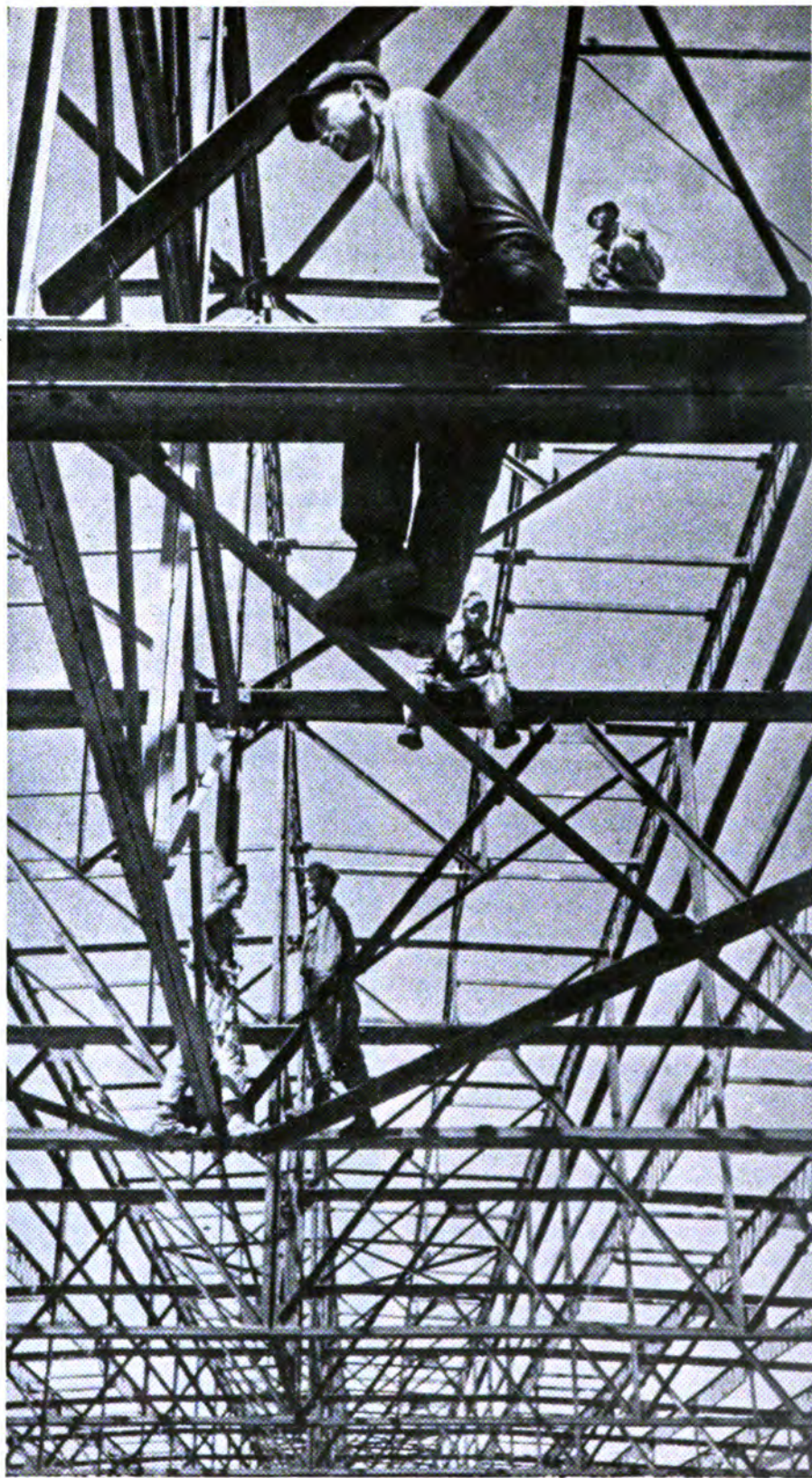
FRAMEWORK. Structural steel workers are building the Kanaker aluminum works, another project resulting from the Sevan hydropower plan.
