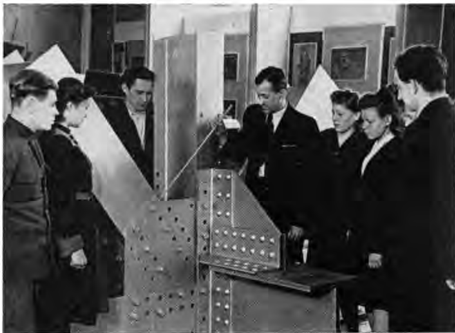
BRIDGE UNIT. A group of visitors inspects a full-size unit of a railway-bridge span.
