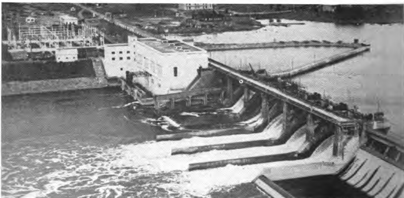
POWER STATION. The Kegum hydroelectric station on the Dvina river in Latvia, wrecked during the war, is substantially restored.
