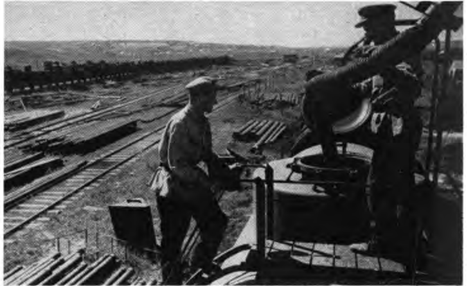
SHIPPING OIL. Pouring petroleum into tank cars at Saratov refinery.
