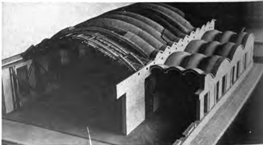
BRICK ROOF. Model of a factory section with thin-walled ribbed brick roofing.
