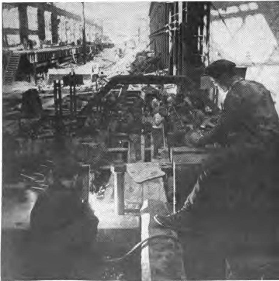
CONSTRUCTION. Welders working on the rebuilding of the Zaporozhstal slabbing mill, one of the world's largest.
