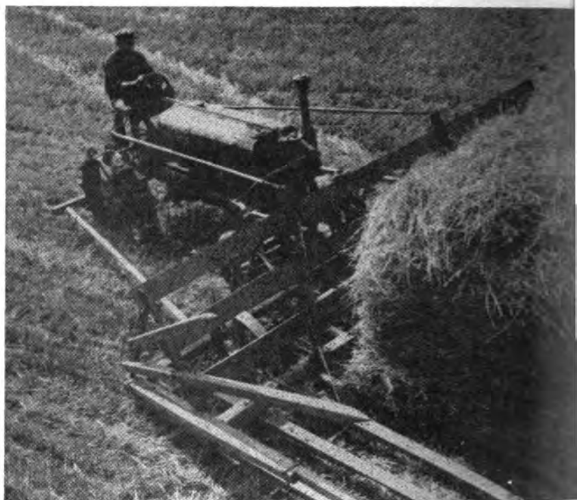
MAKING RAKING EASY. A tractor-driven hay and straw rake designed at the Akimov research station for mechanization of agriculture.
