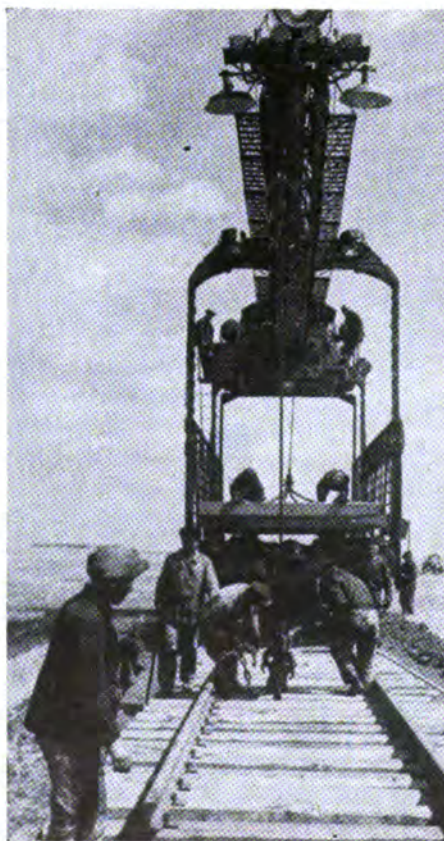
BUILDING. Machines are used for laying ties and tracks.
