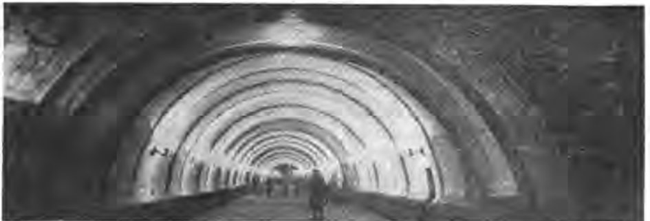
Radiophoto A view of the new subway tunnel connecting the Okhotny Ryad and Ploshchad Sverdlova stations in Moscow. The tunnel is 127 meters long and 7.6 meters wide. Passengers now change from one station to another in three minutes.
