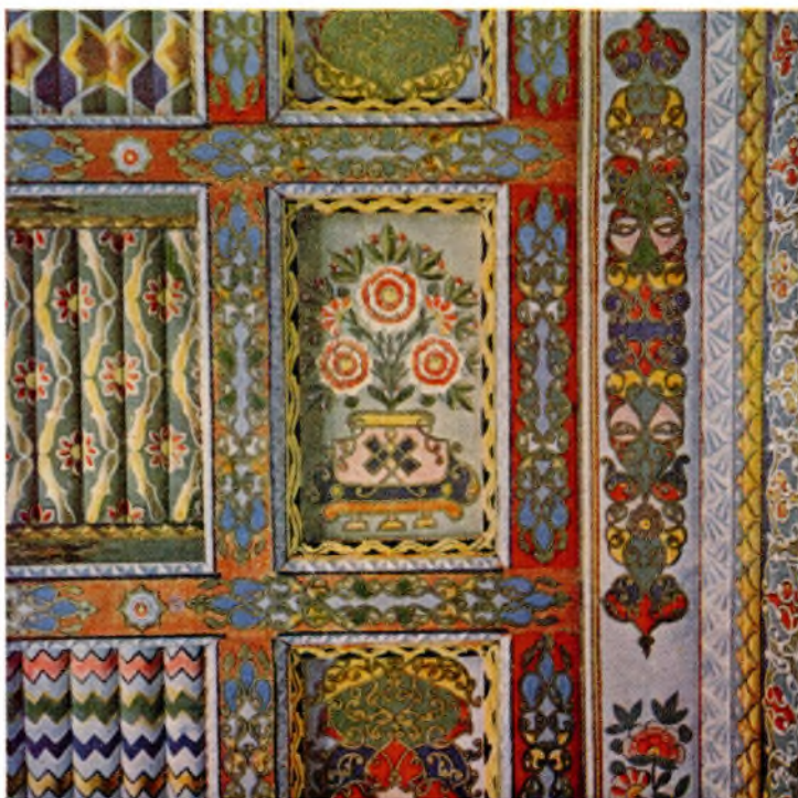
The ceilings were painted in sections on the ground, hoisted aloft and fixed into place. There are no seams or joints evident, however.
