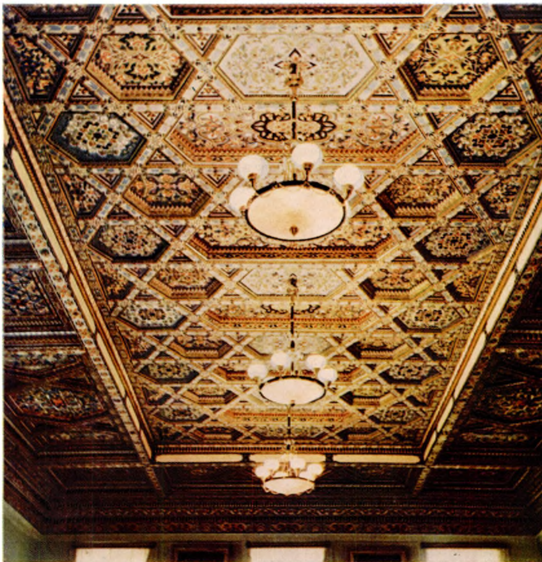
The timbered ceilings made of a series of convex bars worked into one another between the main beams are laid in a variety of geometric designs.
