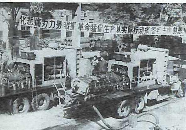
The 1,200-atmosphere fracture trucks made by the Lanchow General Machinery Plant.
