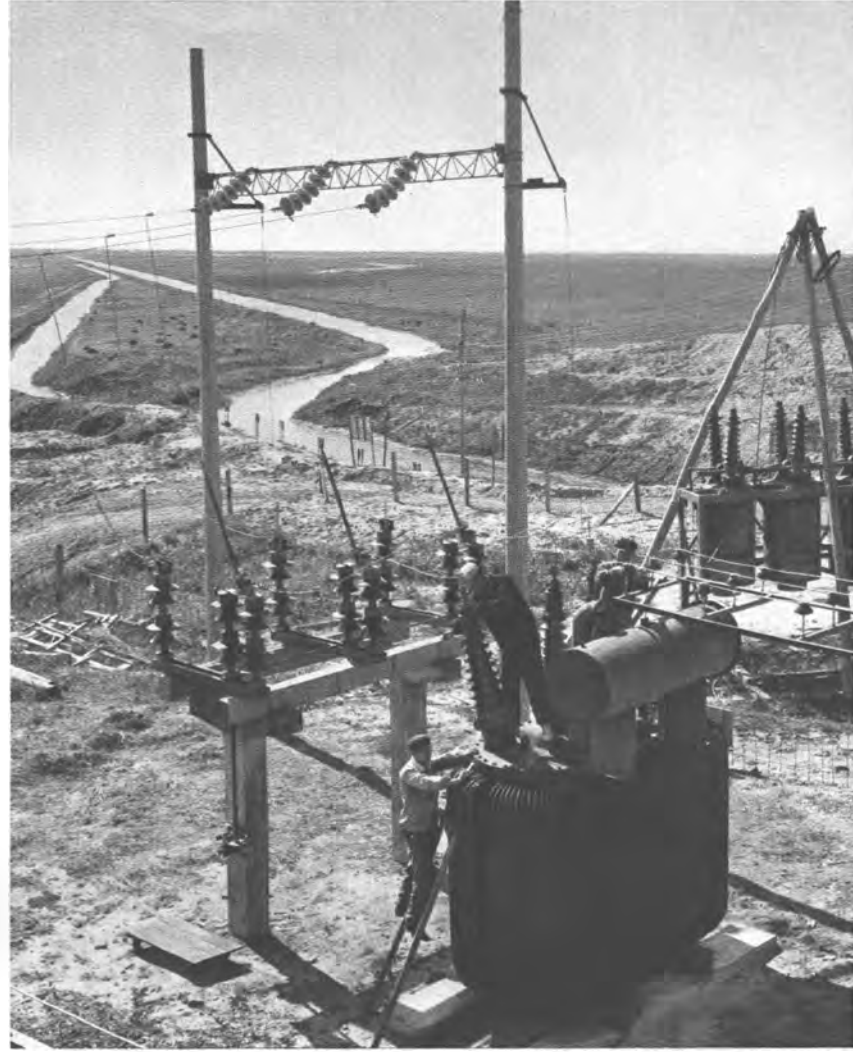
Manufactured by the transformer plant in Chaotung County, the 1,800-KVA transformer has already proved useful in the construction of water conservancy projects throughout the county.
