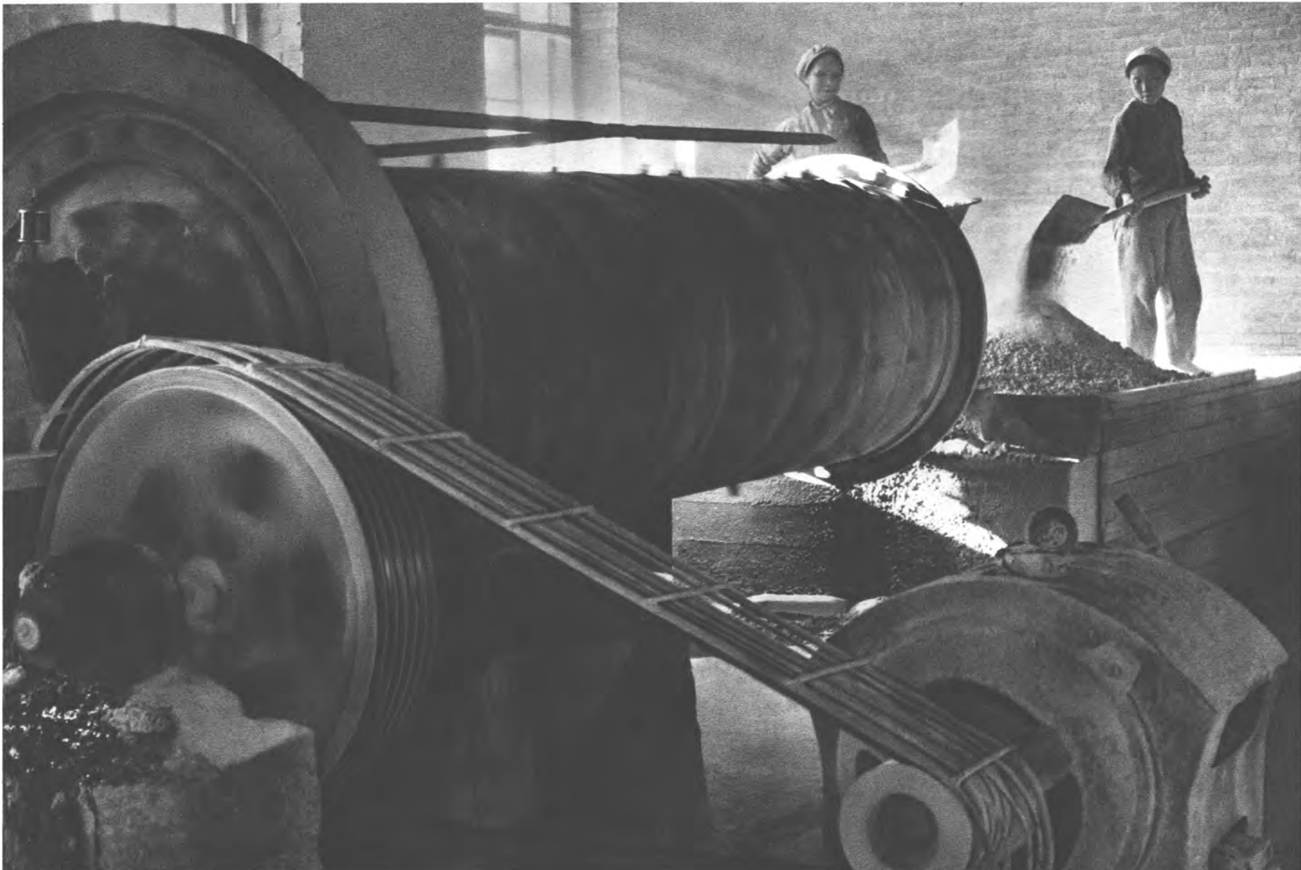
A small-sized cement plant.
