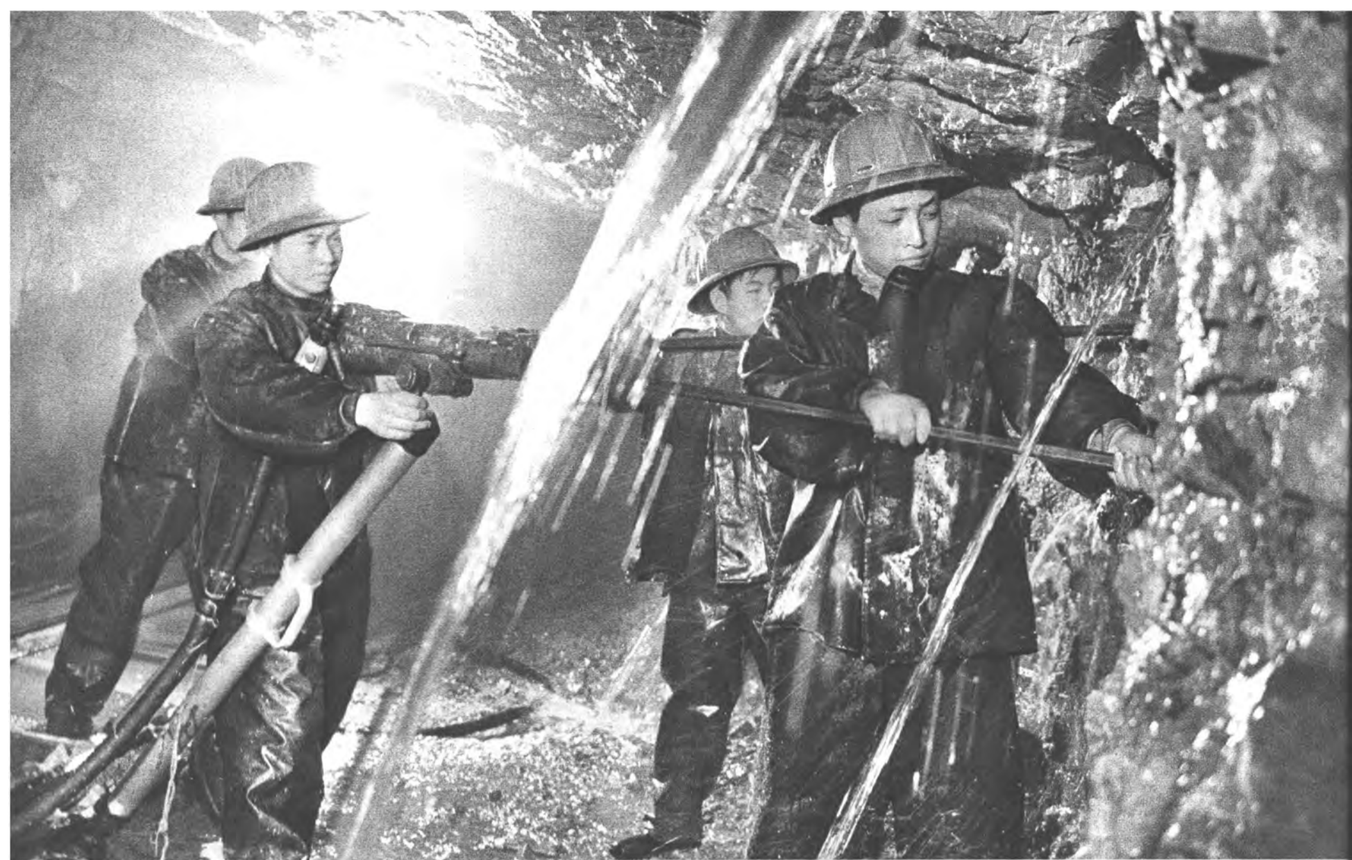
Making a tunnel for the revolution. The greater the hardships, the greater the honour and drive.
