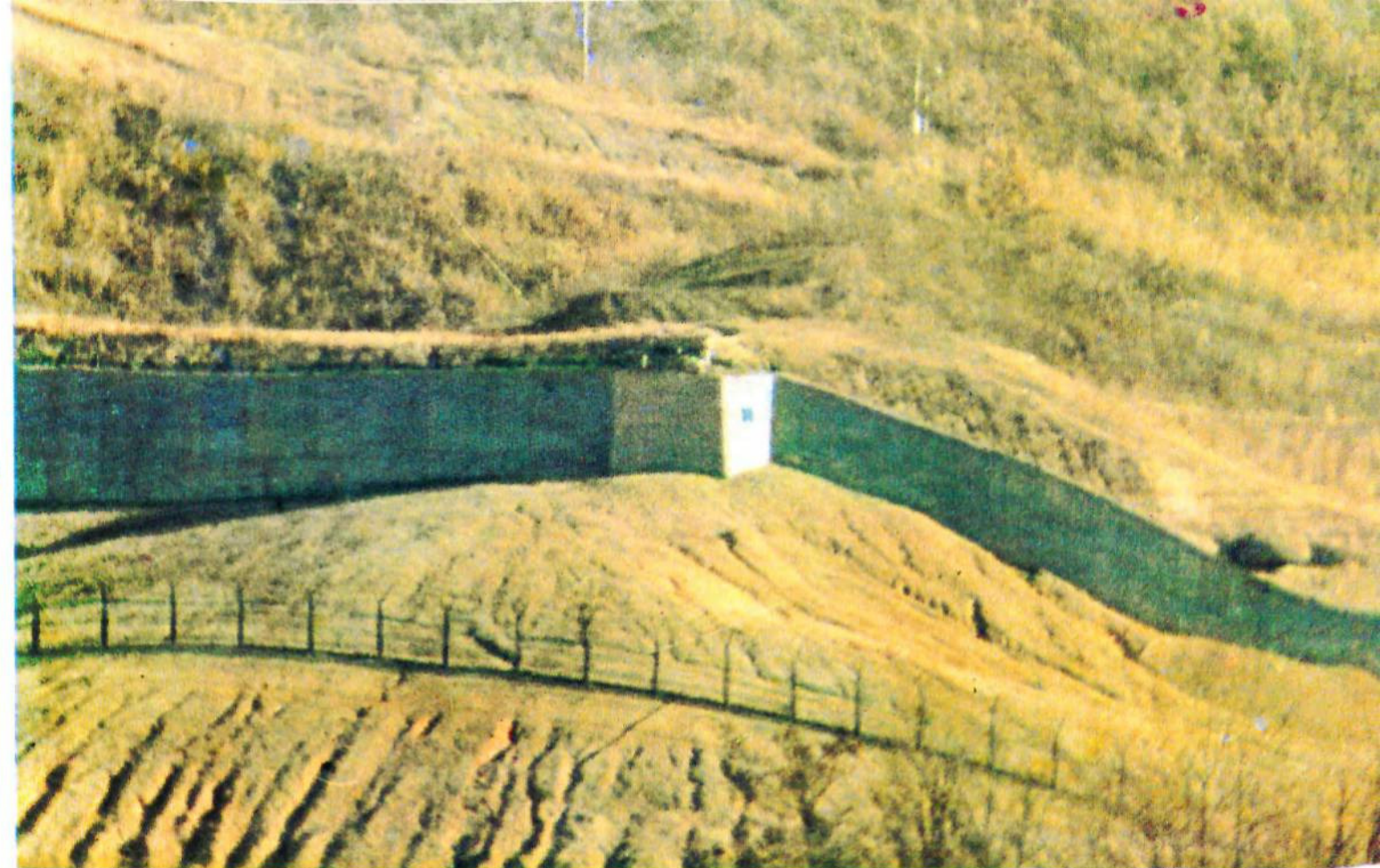
The barrier stretches out over hillocks
