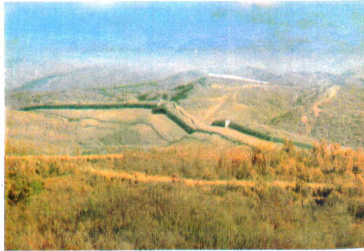
The concrete wall stretches out
