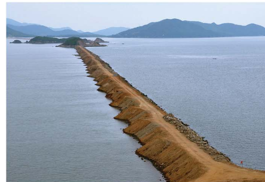
First damming up has been finished at Section 3 in the second stage project of Honggondo tideland reclamation
