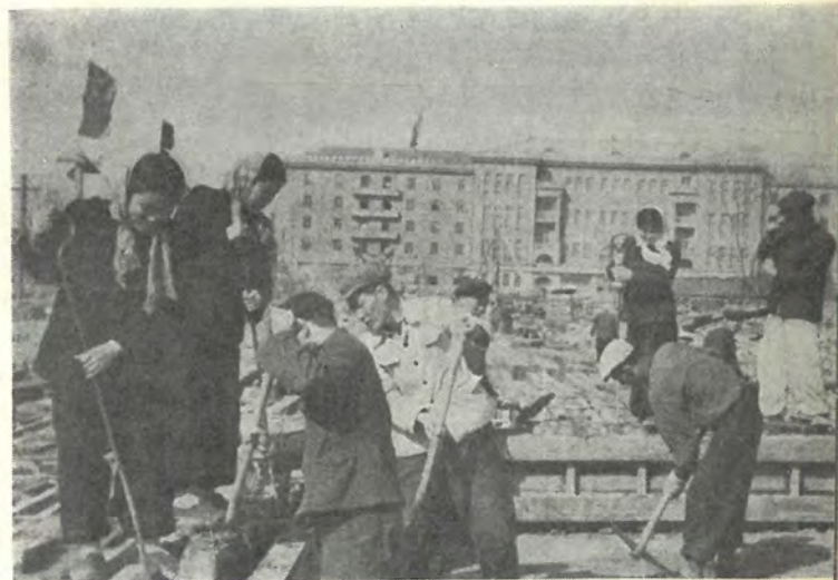
Government workers are helping with construction
