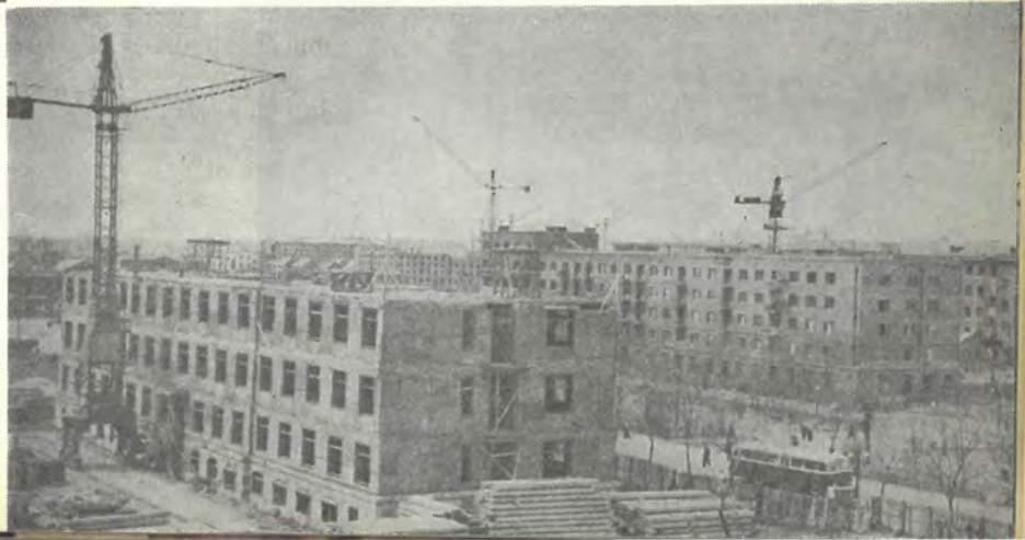
Prefabricated houses under construction
