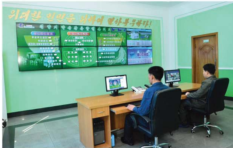
The integrated control office.
