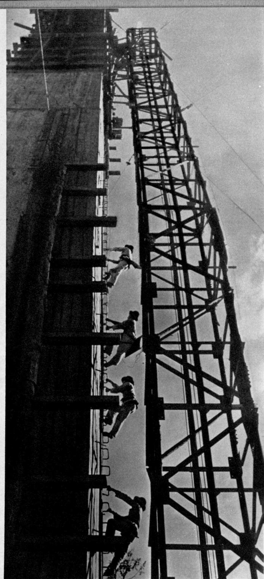
A 60-metre pier under construction.
