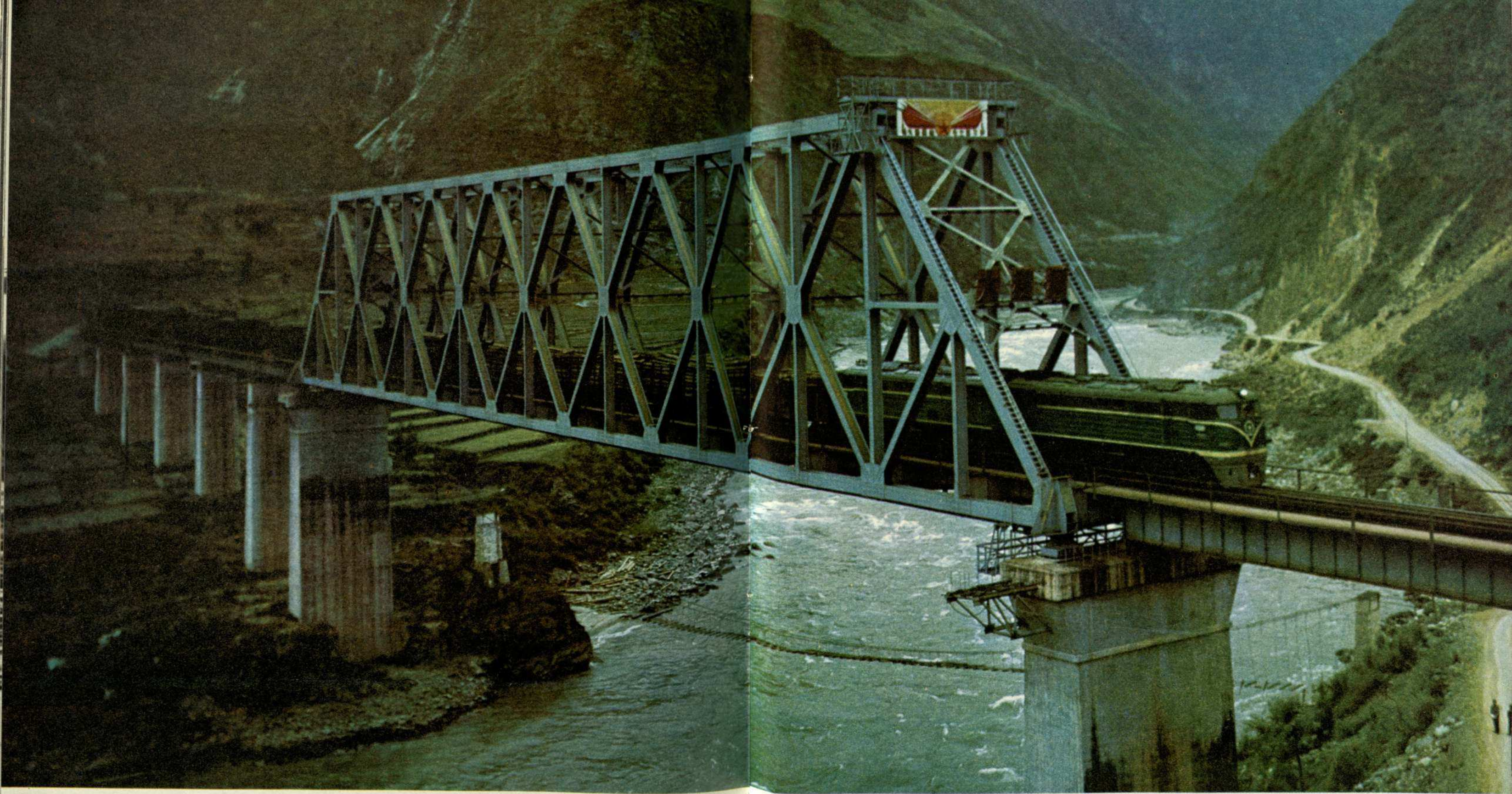
This railway bridge stretches across the lower reaches of the Tatu River, while spanning its upper reaches is the Luting Iron Chain Bridge on which the Red Army crossed during its Long March.
