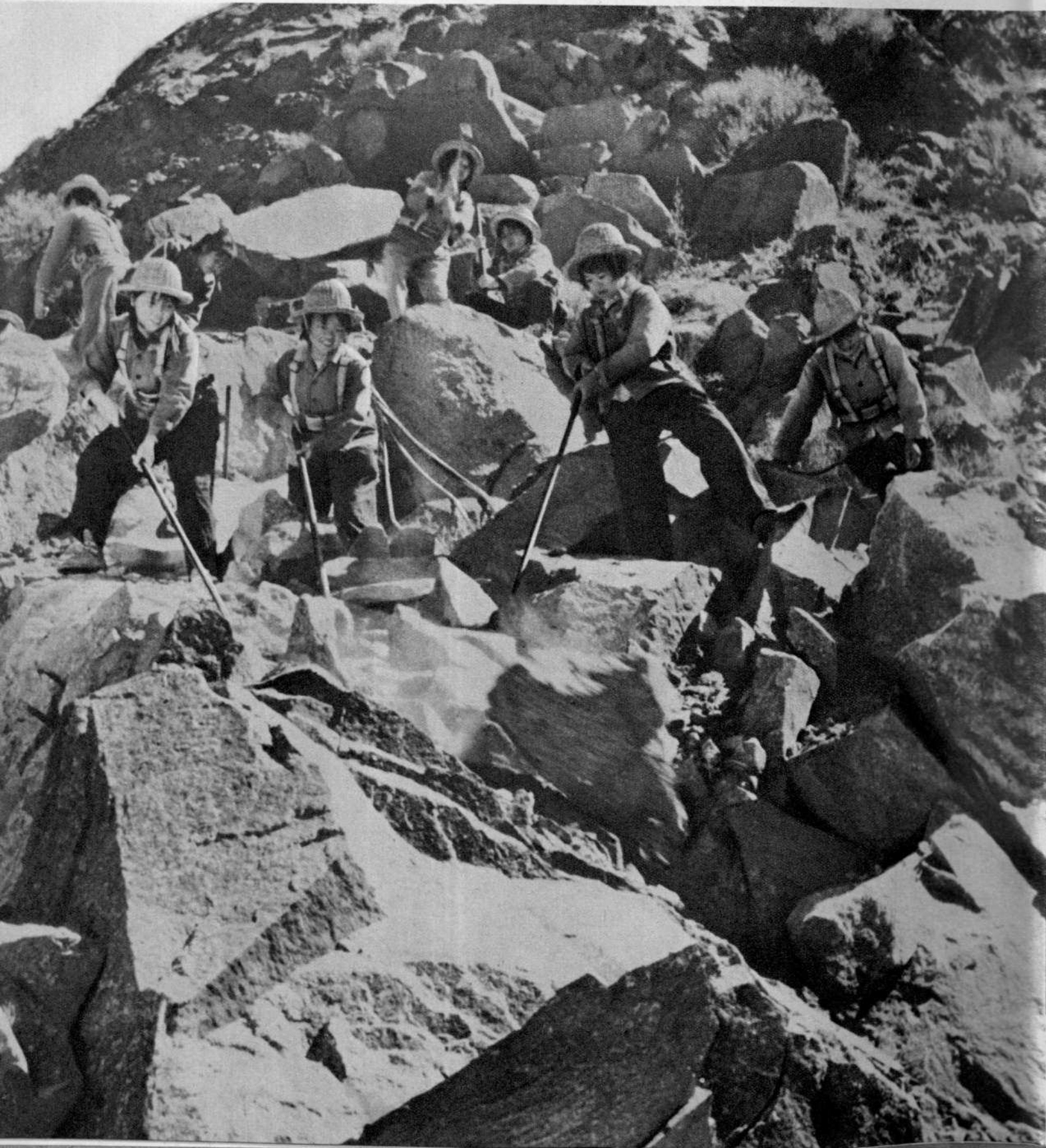
The project received the active support of the local people. Militia women here take on a job of quarrying rock.
