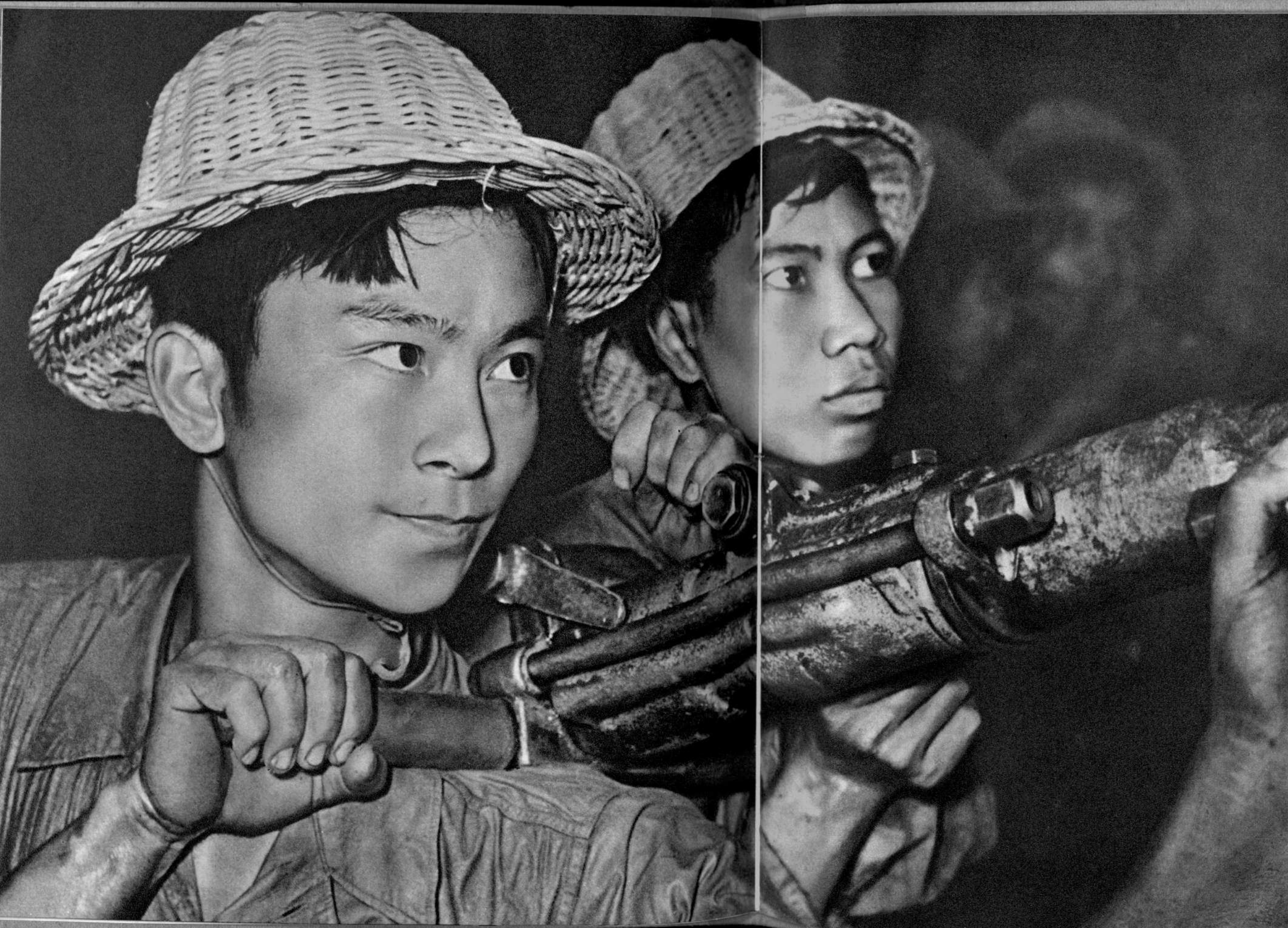
Complex geological conditions made the round-the-clock work of tunnelling extremely difficult, and the intrepid railway builders exerted untiring efforts to accomplish the task.
