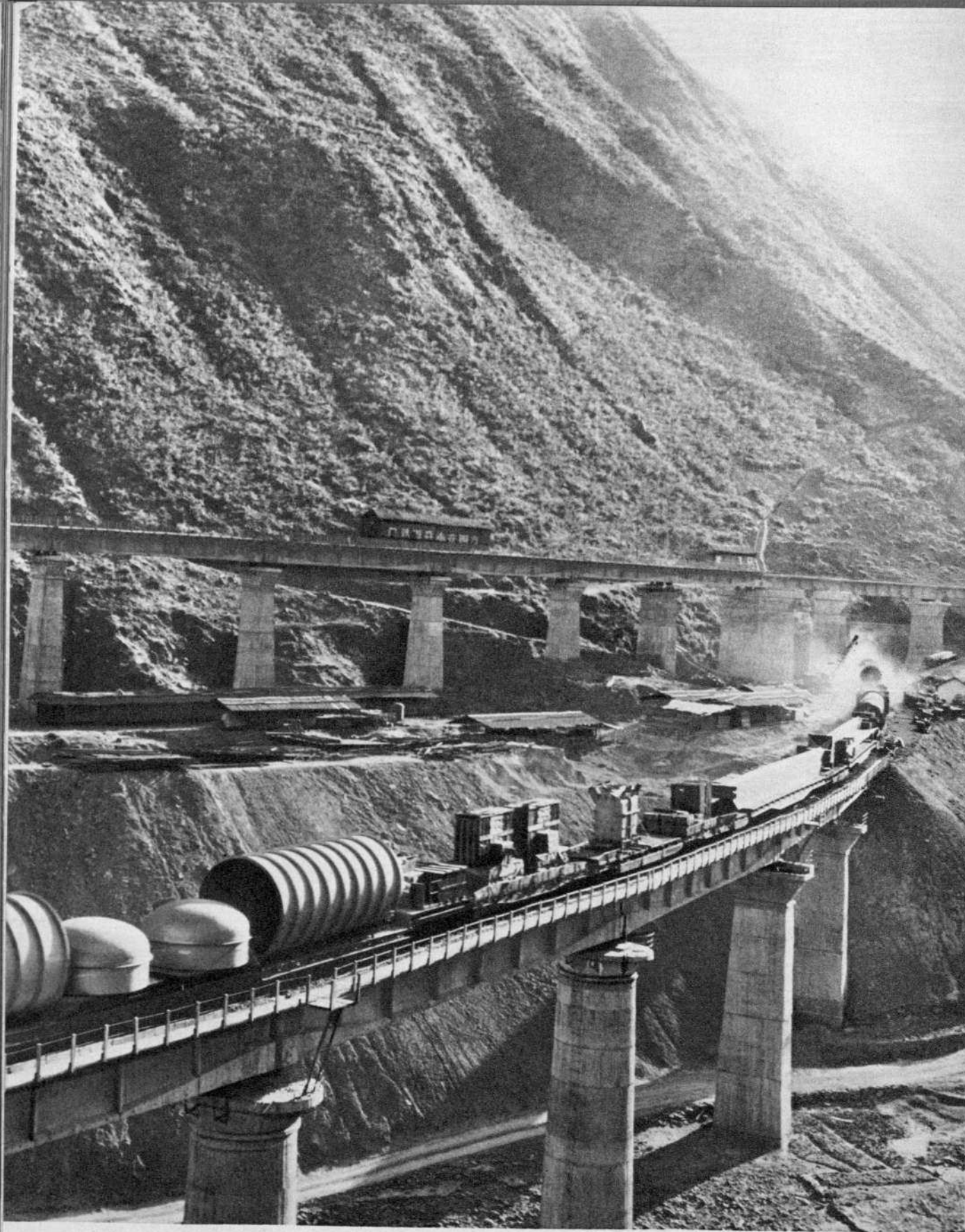
A goods train loaded with construction materials winds its way along the route.
