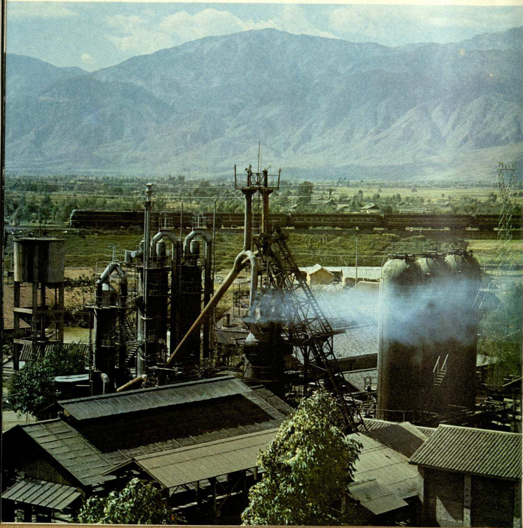
A small iron and steel plant built recently beside the railway.
