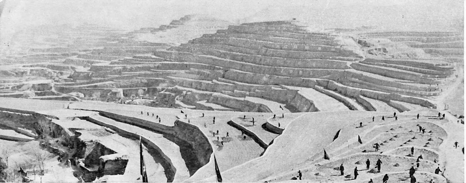
Extensive terraced fields control loss of water and soil along the upper reaches of the Yellow River in Kansu province.
