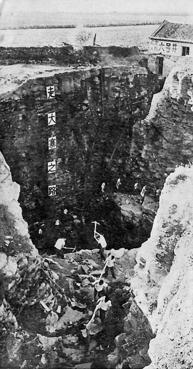
Sinking a well.
