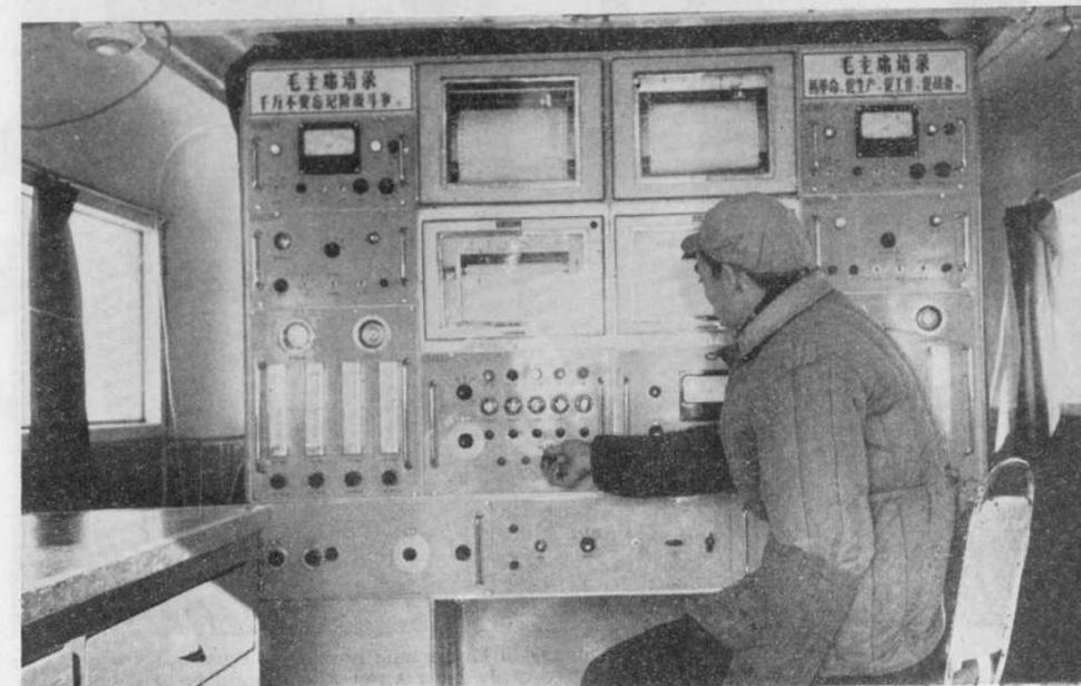
A worker operates the automatic gas chromatograph designed and made by the Taching workers with the help of brother industries.
