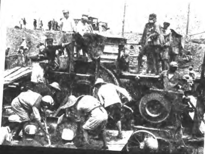
PLA men operating concrete mixers.
