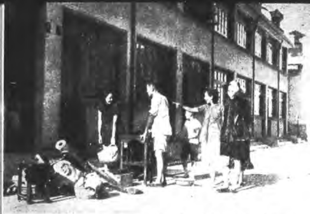
A five-lane slum on Shanghai's Canton Road was recently torn down and rebuilt at government expense. Photo shows working class families moving into the new apartments.
