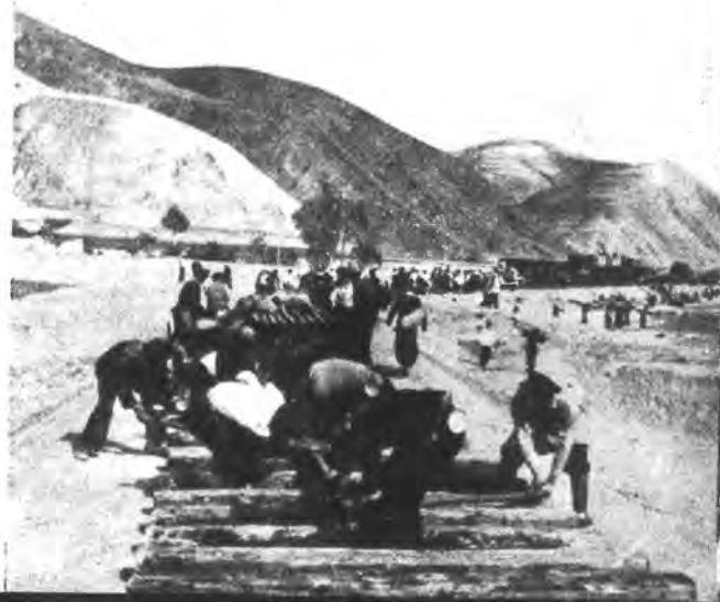
Laying ties at high speed.
